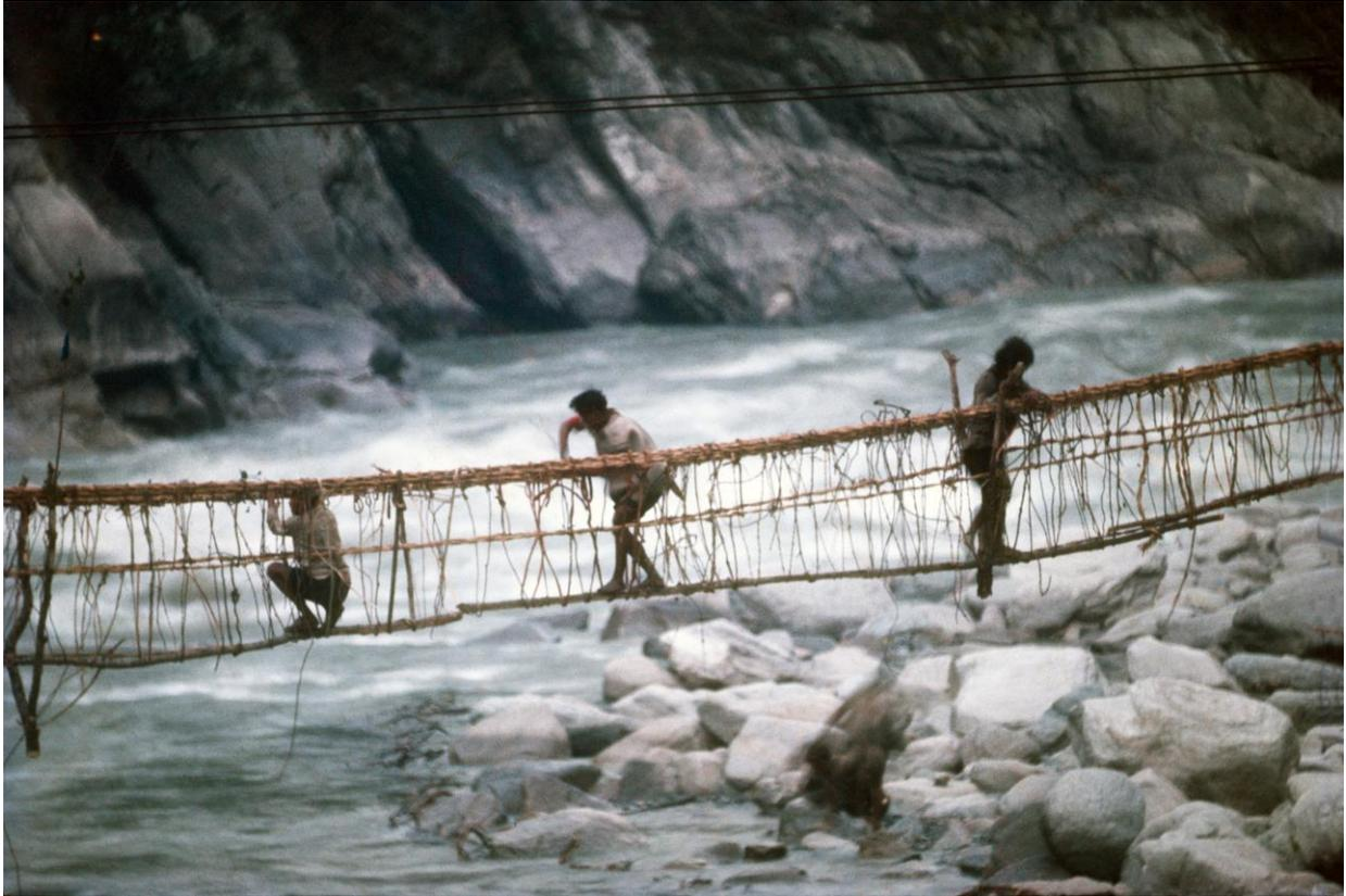
**Figure 3.** The bridge made of woven vines over the Arun below Num, being repaired and upgraded by porters prior to its crossing by more than 285 porters, each carrying an 80-pound (36 kg) load (photograph by J. McNeely).
