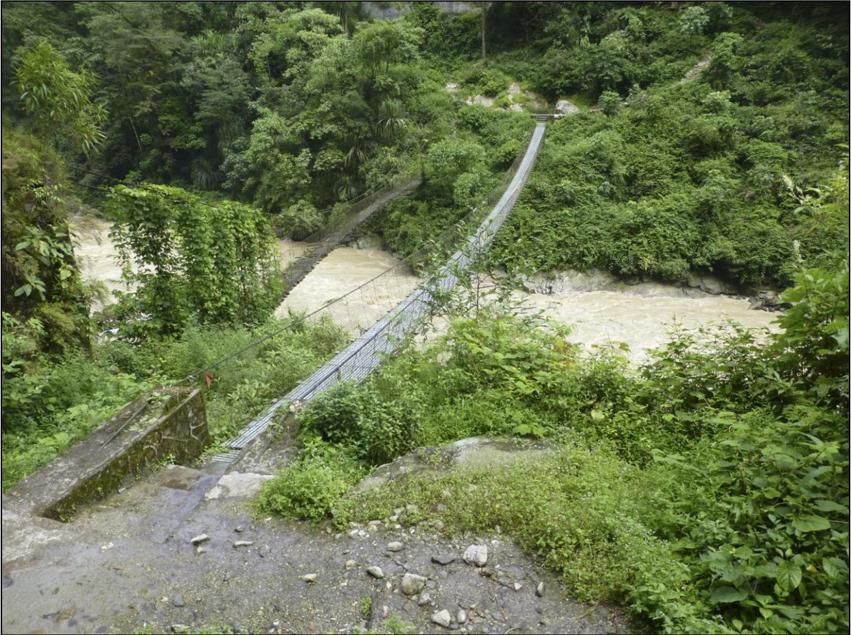
**Figure 4.** The metal cable bridge today. The old wooden bridge which replaced the bamboo and rope bridge of the 1970s can be seen to the left, or downstream, of the new metal cable bridge (photograph by A. Byers).
