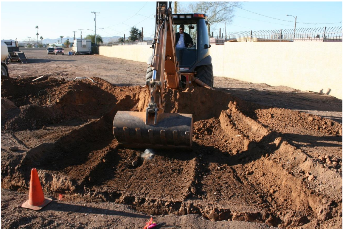
Figure 2. Stripping the Overburden at an Archaeological Site with a Backhoe Stripping Bucket.
