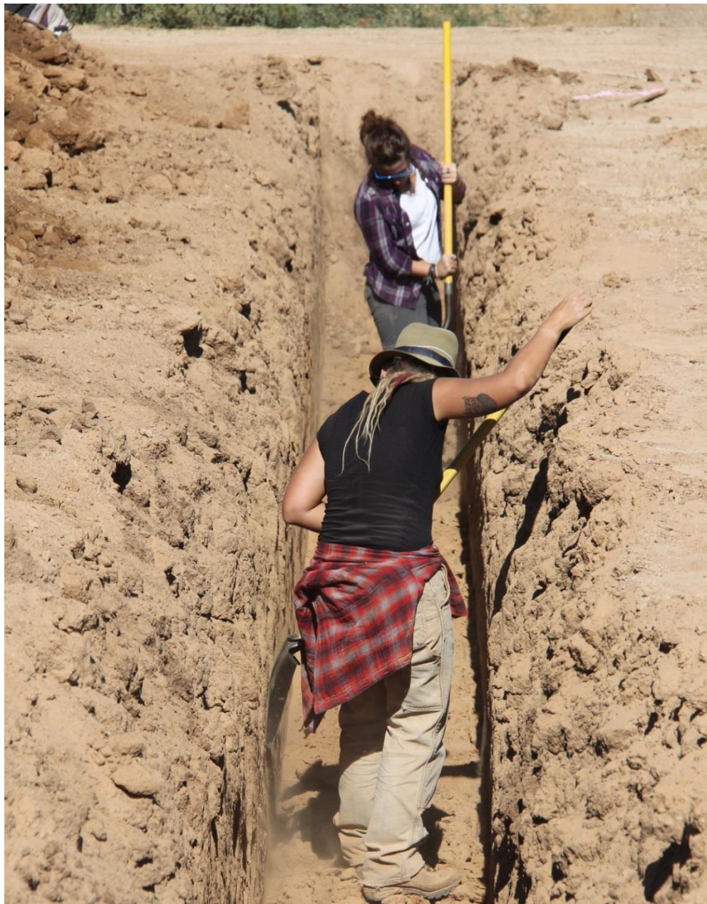
Figure 1. Cleaning the Side-walls of a Backhoe Trench with Shovels.
